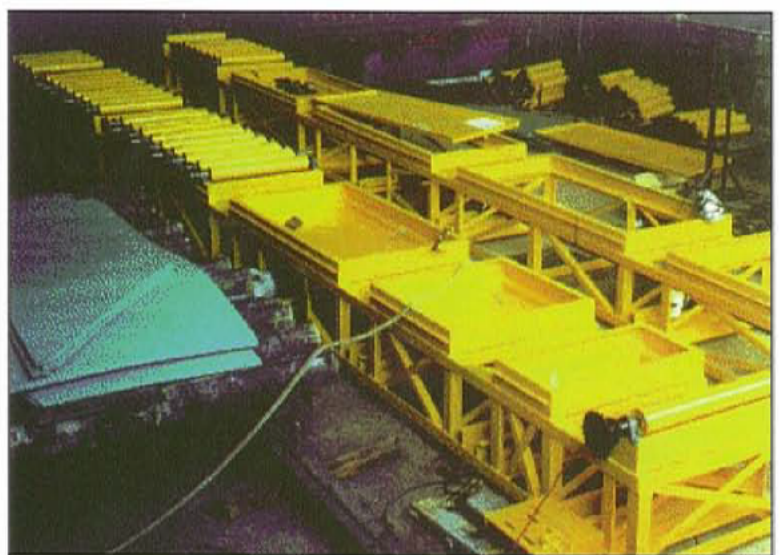
ASSEMBLING ROLLS TO CONVEYOR FRAMES
