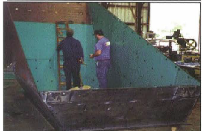
SCREEN CHUTES BEING LINED WITH UHMW
